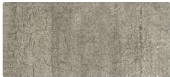
CN 6481 P Cement Concrete
